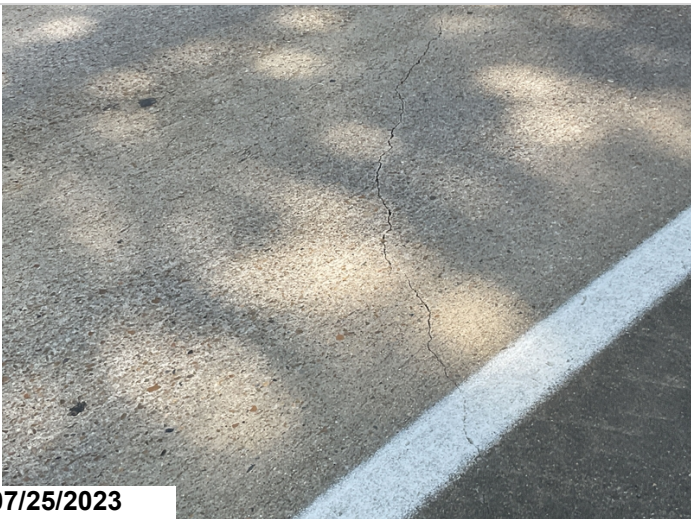
Span 2 deck right has large unsealed cracks.
