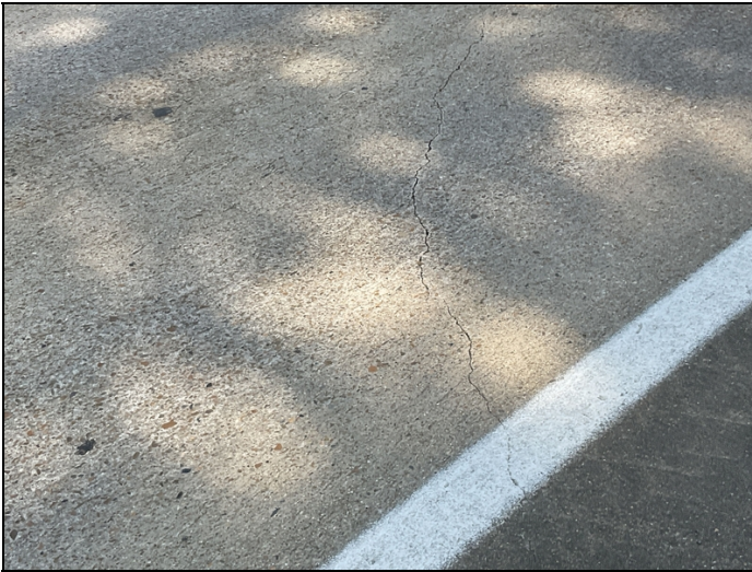
Span 2 deck right has large unsealed cracks.
