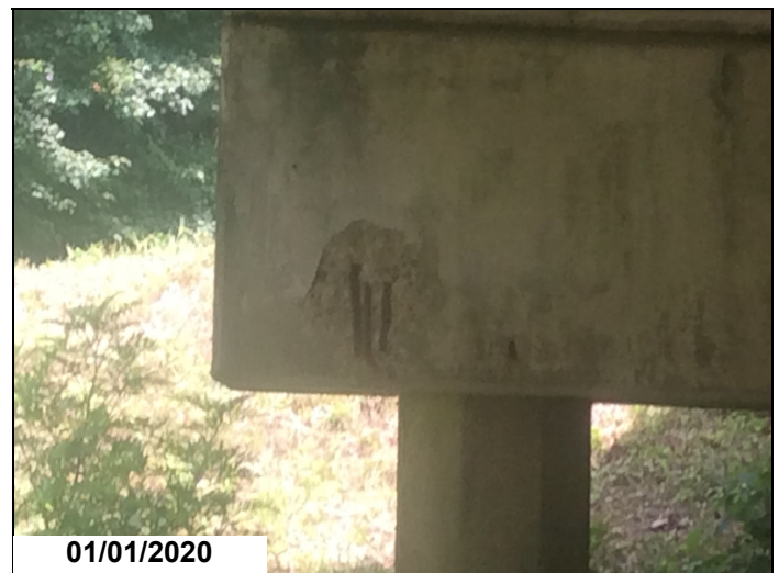
Bent 3 cap left has spall with exposed rebar.
