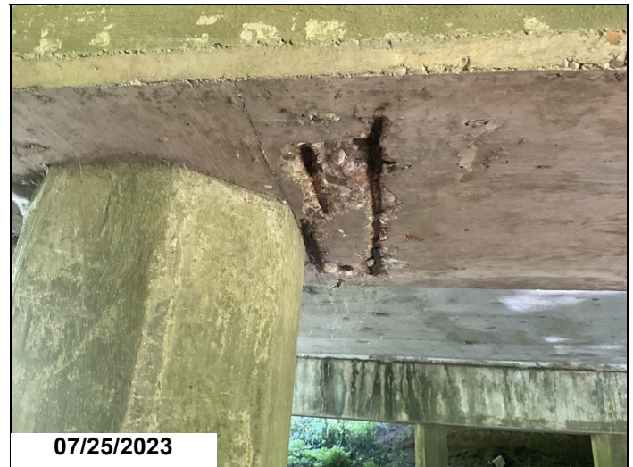
Bent 2 cap near pile 2 has spall with exposed.
