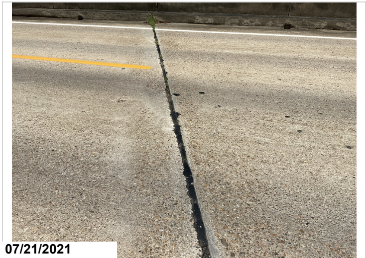
Bent 2 joint seals have lost bond with areas missing.
