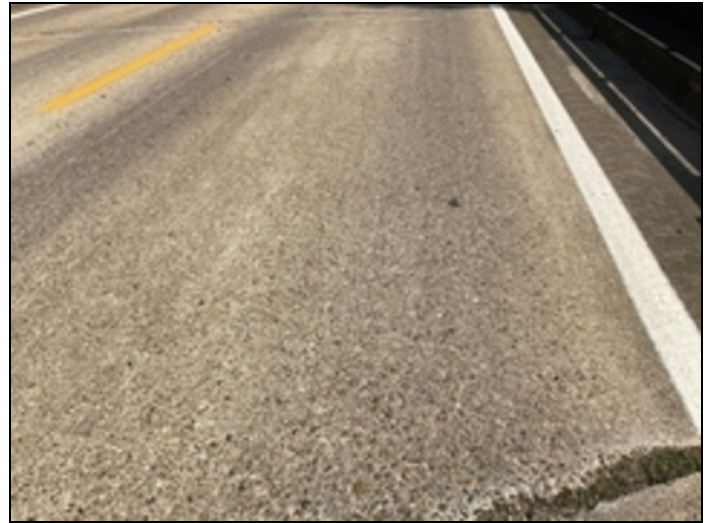
Span 1 deck right has large unsealed cracks.
