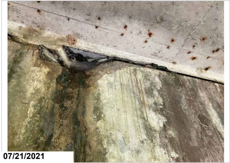
Bent 3 right key way in cap has spall with exposed rebar.
