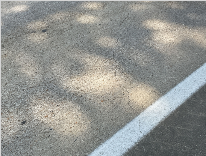
Span 2 deck right has large unsealed cracks.
