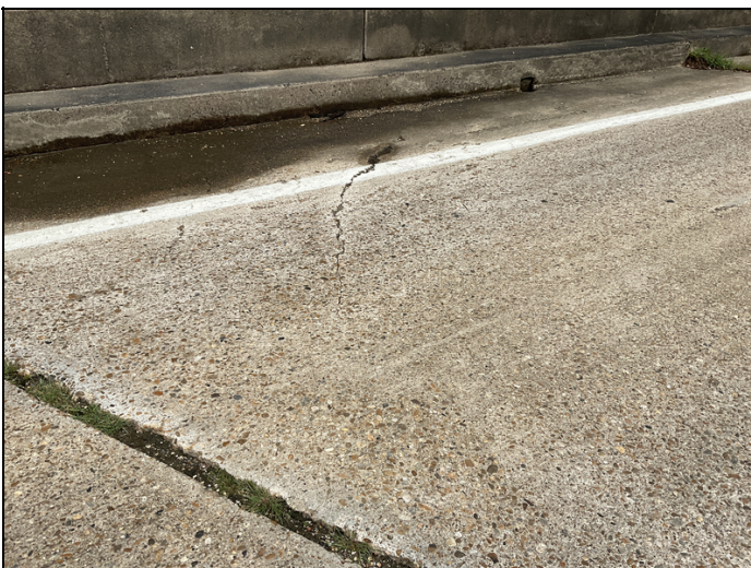
Span1 left has large diagonal crack.
