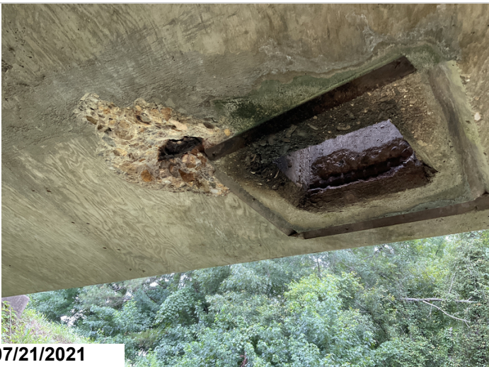
Span 3 right has soffit spall near drain opening.
