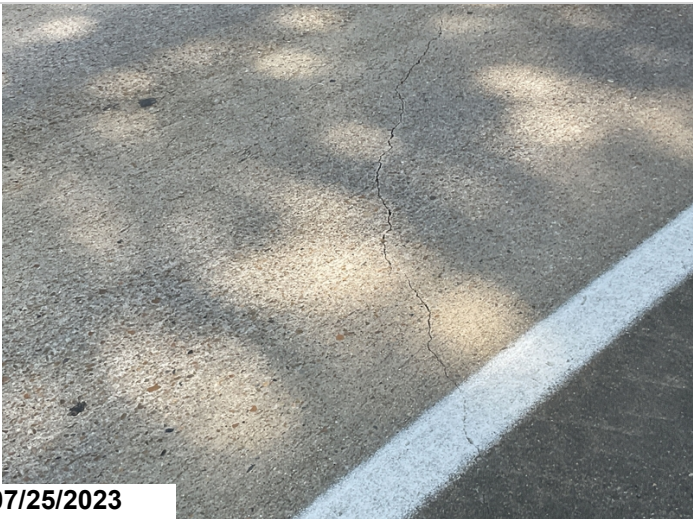
Span 2 deck right has large unsealed cracks.
