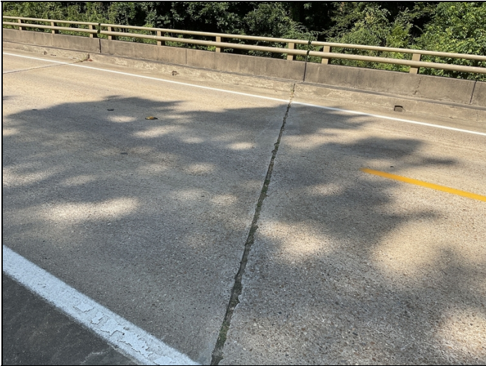
Bent 3 joint seal has loss of adhesion and is missing.
