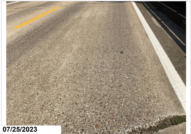
Span 1 deck right has large unsealed cracks.
