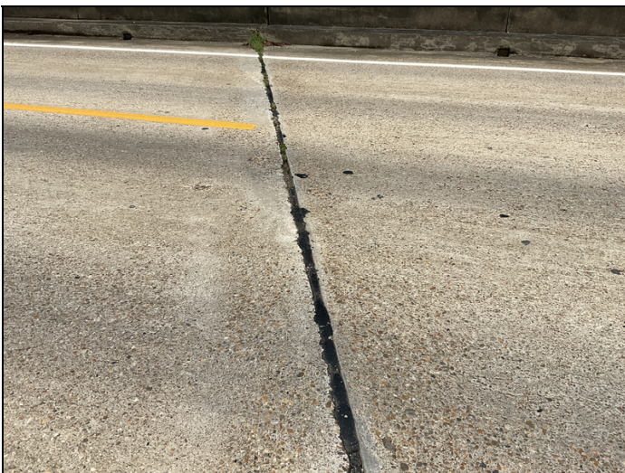
Bent 2 joint seals have lost bond with areas missing.
