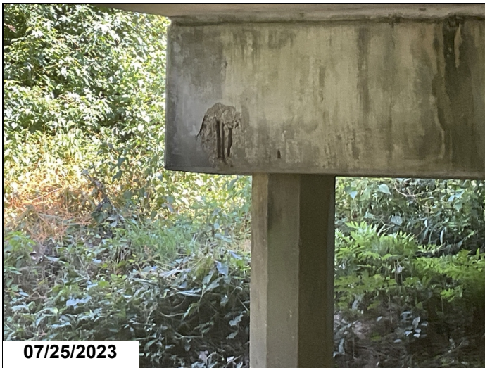
Bent 3 left ahead near pile 1 has spall with exposed rebar.
