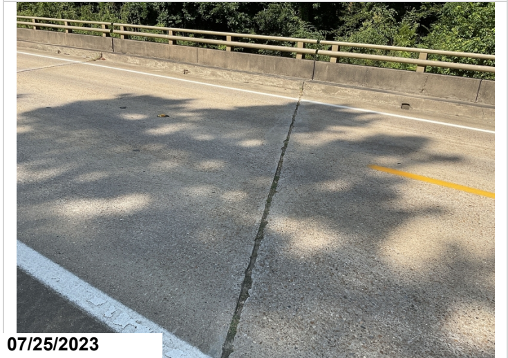
Bent 3 joint seal has loss of adhesion and is missing.
